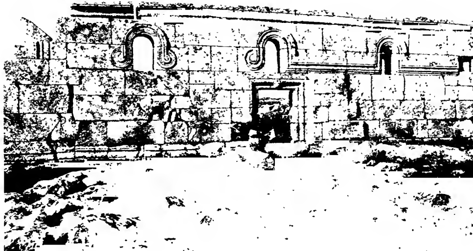
South wall of South Church at Dār Kitā.
